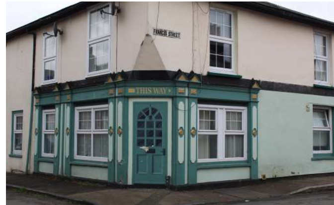
Figure 46 Historic shopfront on Sydney Street
