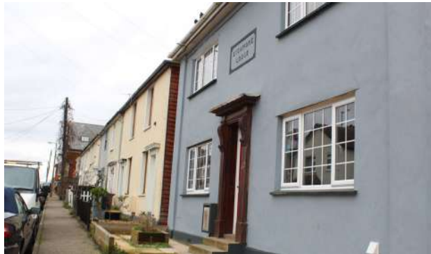
Figure 76 Row of terraces from 42 John Street
