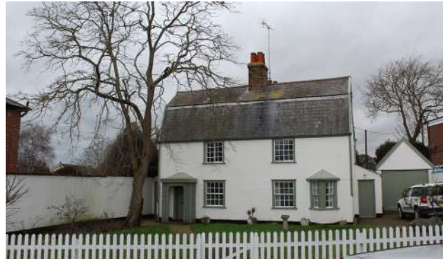
Figure 65 Grade II Listed Lower Green Cottage
