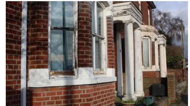
Figure 25 Architectural detailing of houses on Hurst Green
