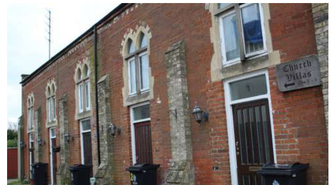
Figure 79 Former Congregational Chapel
