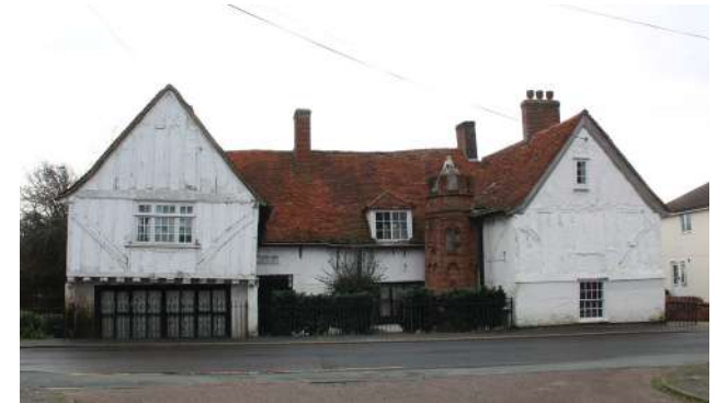
Figure 33 Grade I Listed Jacobes Hall
